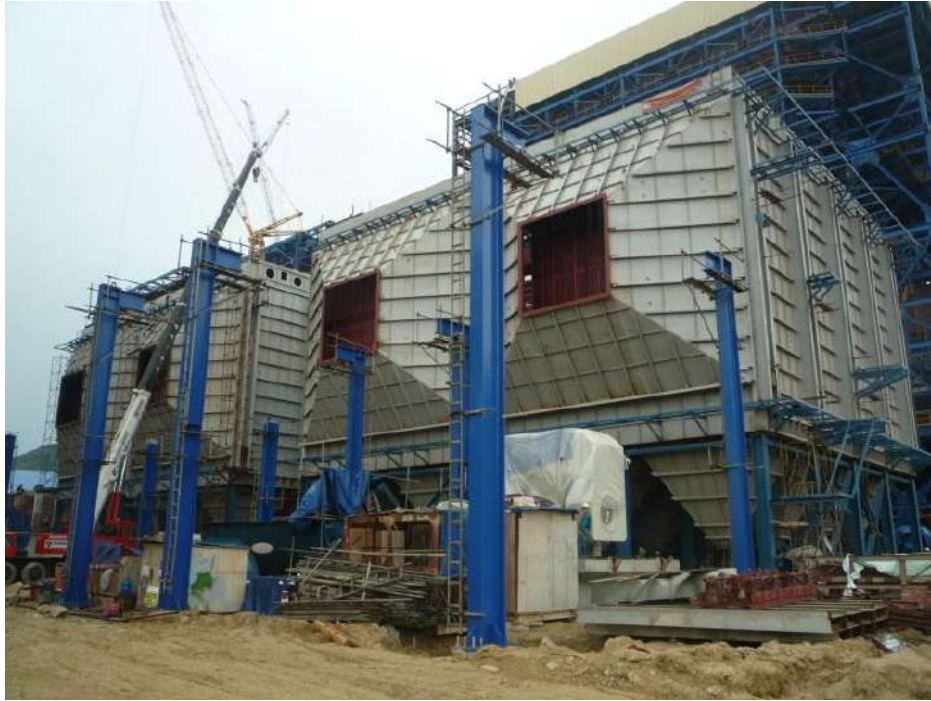
ESP before thermal insulation
